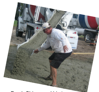
Frank Chivas and his team lay new concrete
