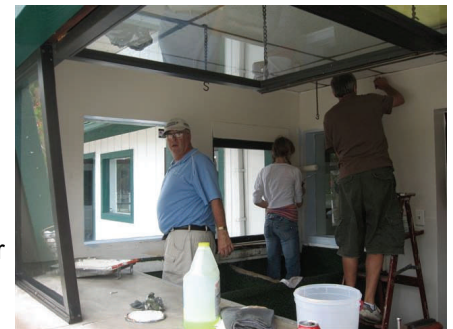
Renovations continue at the Driving Range
